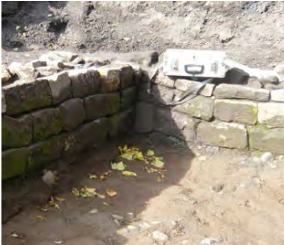
Fig. 13: Roman masonry at Crammond.
