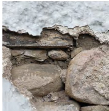
Fig. 19: Earth mortar concealed behind lime finishes.
