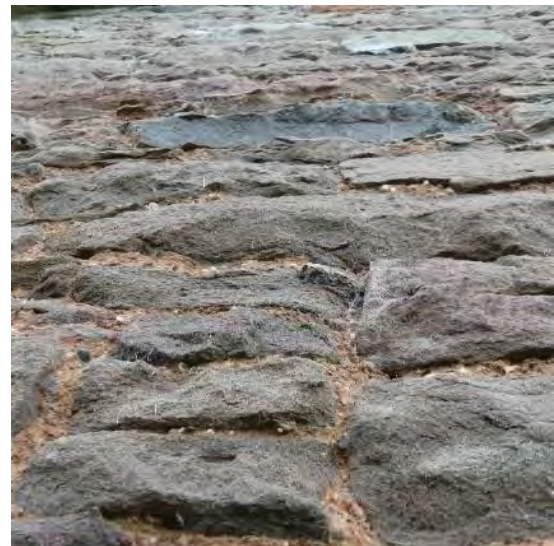
Fig. 11: Detail of earth-lime mortar.
