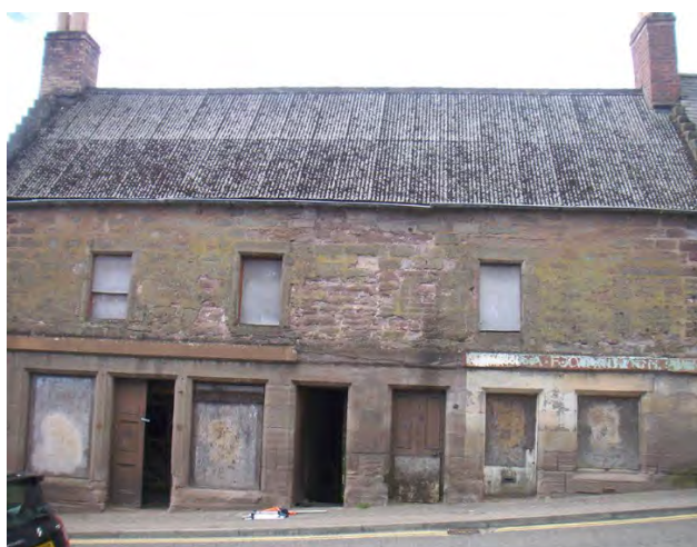
Fig 16: 19 th C. building, Brechin
