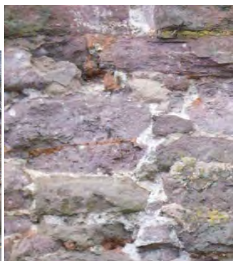
Fig. 17: Earth mortar core, lime pointing
