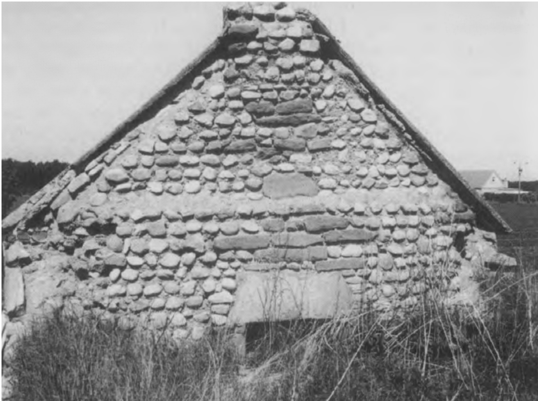
Fig. 9: Clay and Bool wall, Cowfurach, Moray. © HES. Similar arrangements of round river stones laid in herring-bone rows can be found in other countries.
