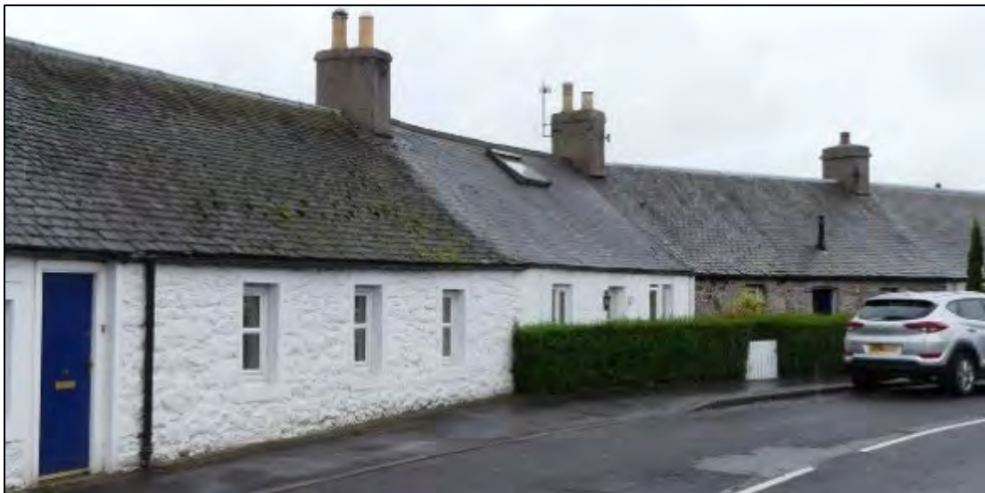
Fig. 15: The village of Longforgan was ‘built with turf and stone or clay for mortar, and not a vestige of lime’ before 1777 (OSA). Soon after, all were replaced by the landowner with smarter buildings, built of earth mortared masonry pointed in lime. See Figs 5 & 6.
