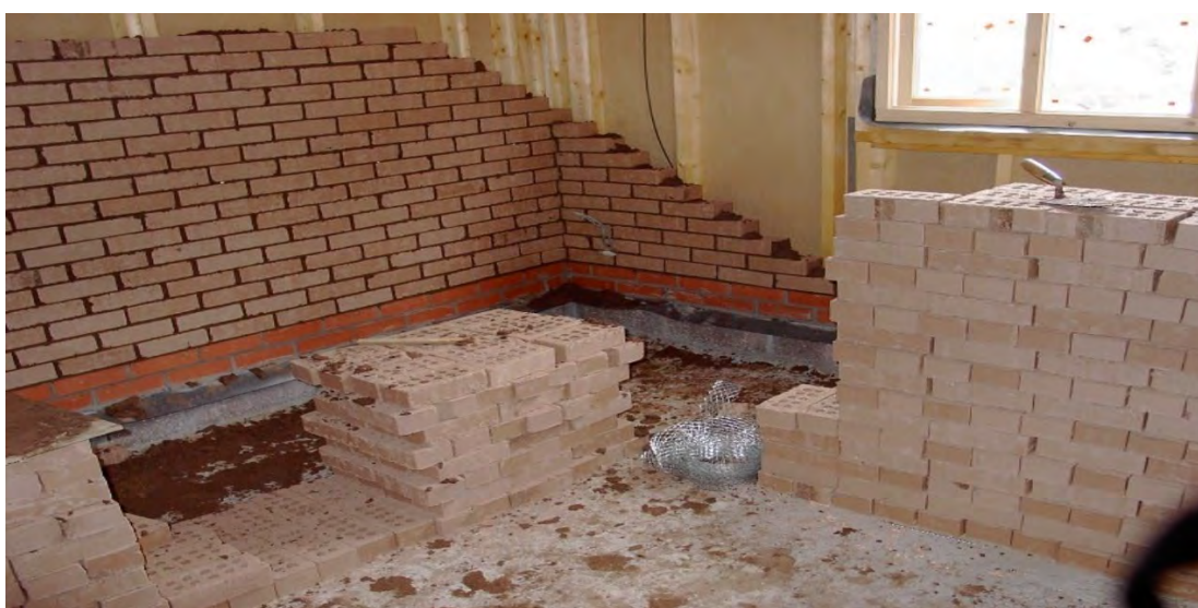
Fig. 22: Earth mortar in contemporary eco-house, Perthshire.
